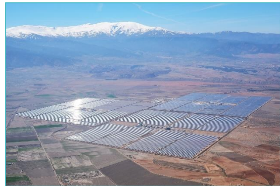
Figure 14: The 150 MW Andasol solar power station in Spain is a parabolic trough solar thermal power plant that stores energy in tanks of molten salt so that it can continue generating electricity when the sun is not shining
